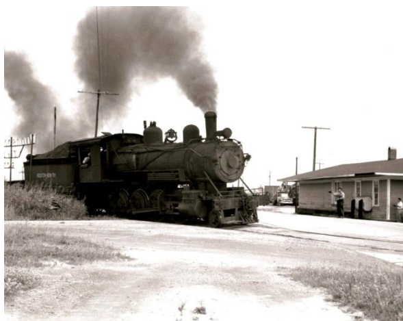
No. 712 at Rt. 34 in Rockton. Station burned in the 1980s.
