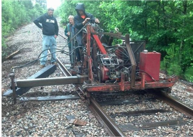
The track crew uses the inserter to place a new tie under the rails.
